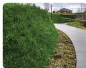
⑤ Reinforced earth / green wall
