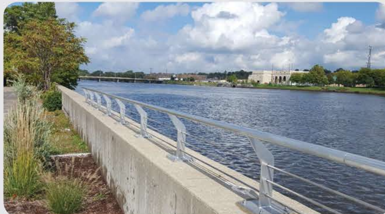
Railing System - 2018 installation at Grand View Place
