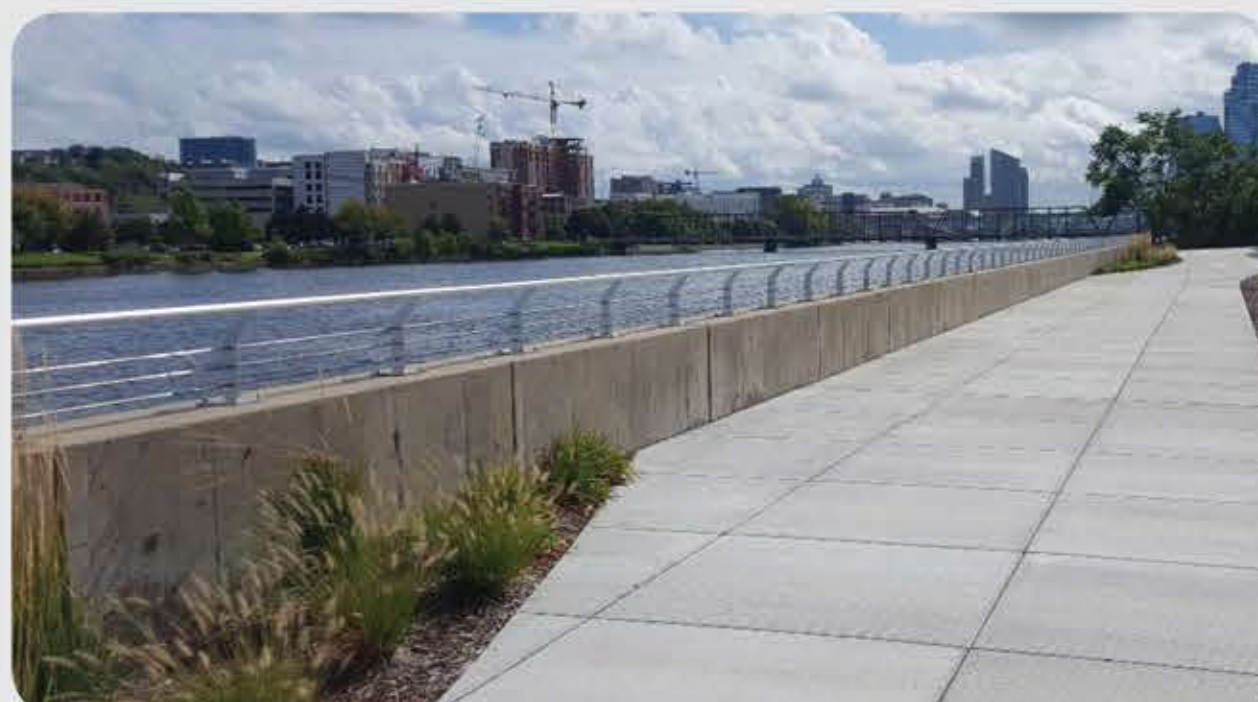
Railing System - 2018 installation at Grand View Place
