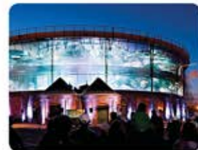
4 Repurposed water tank
